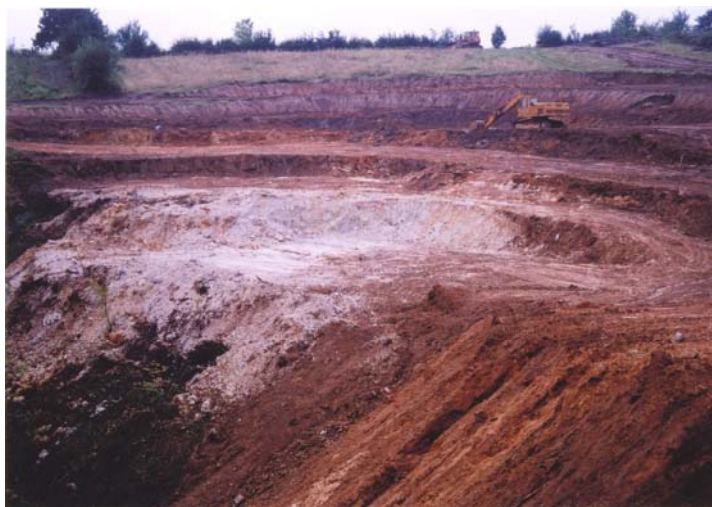
Fig. 1. Surface excavation site of Zorka brick clay Sabac
