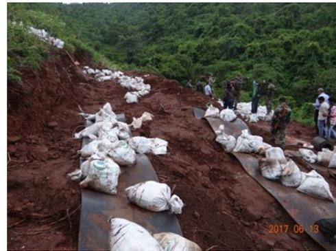
**Figure 4** View of blasting face covered with conveyor belts and sand bags (Blast TB-1)
